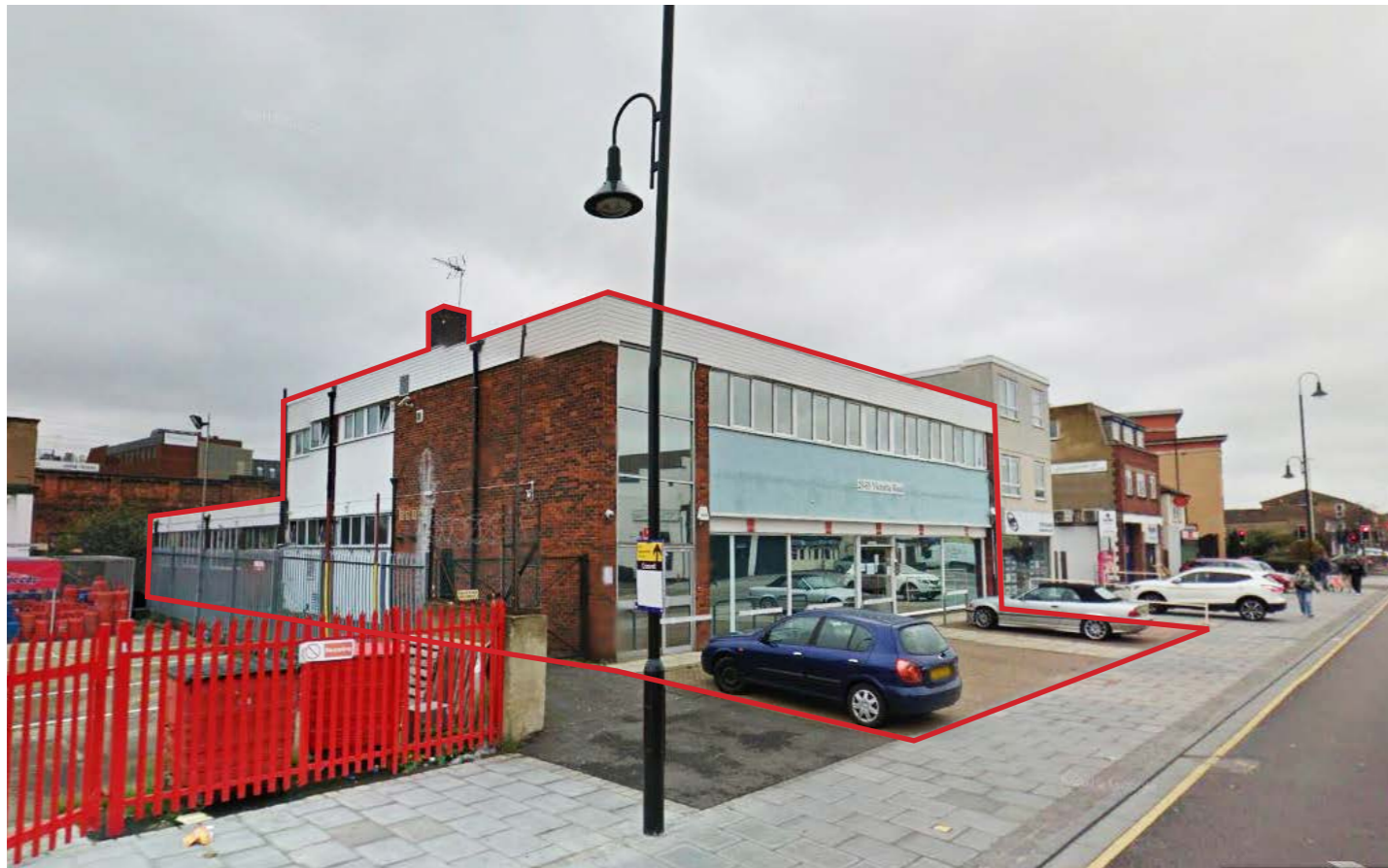
3. View of the site from Victoria Road
