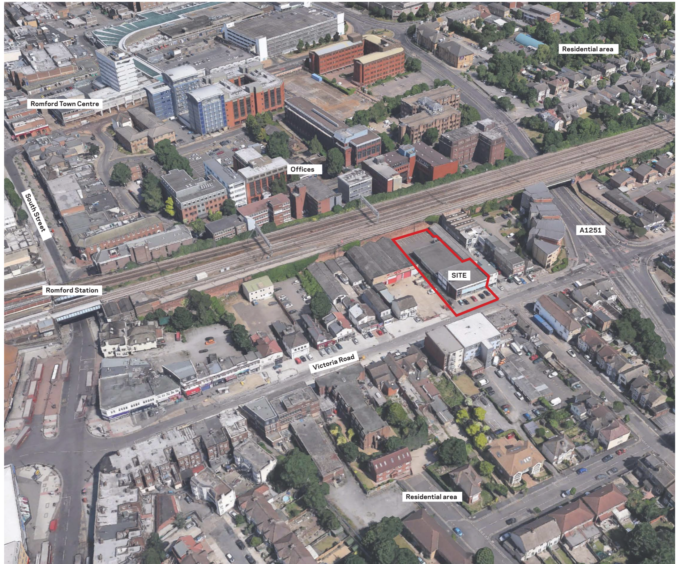
Aerial view of the site
