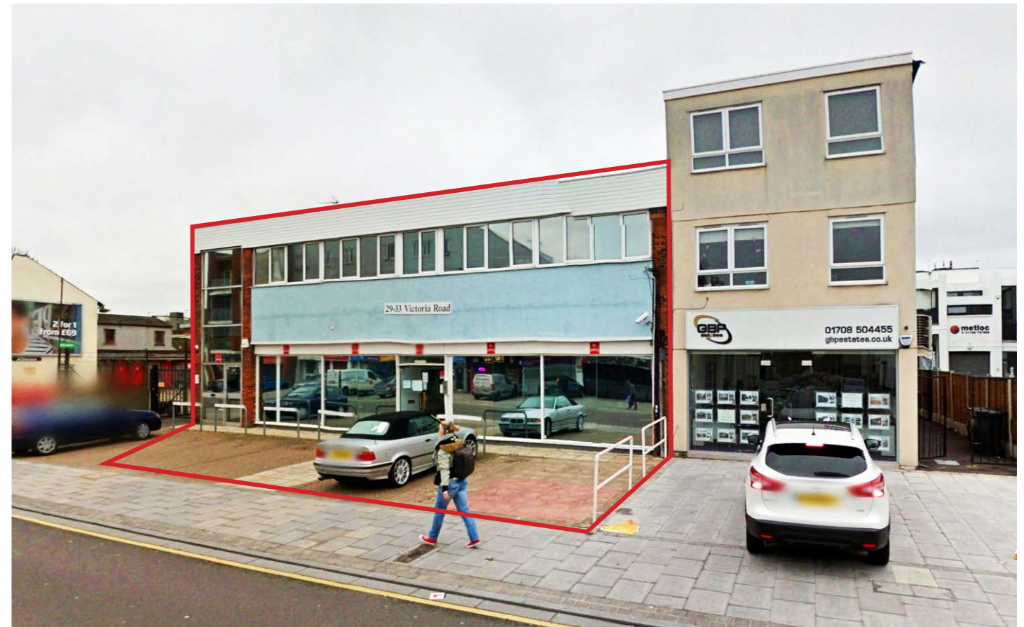
4. Alternative view of the site from Victoria Road
