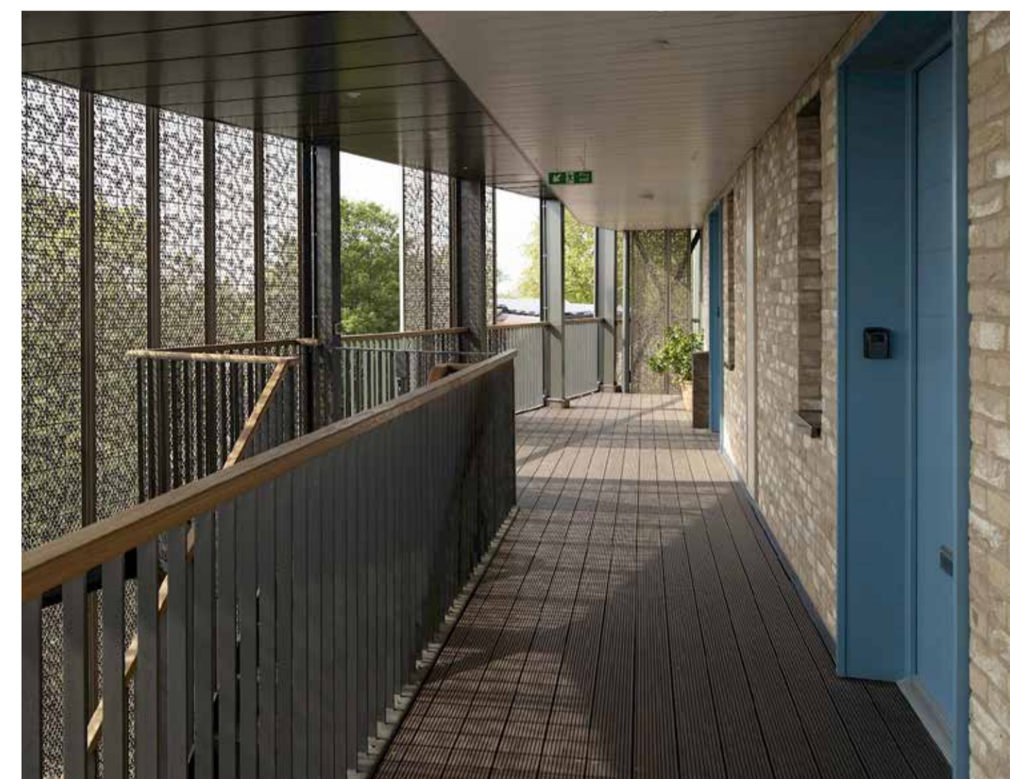
5 - Example of a residential development with perforated metal panels to screen the communal circulation zones
