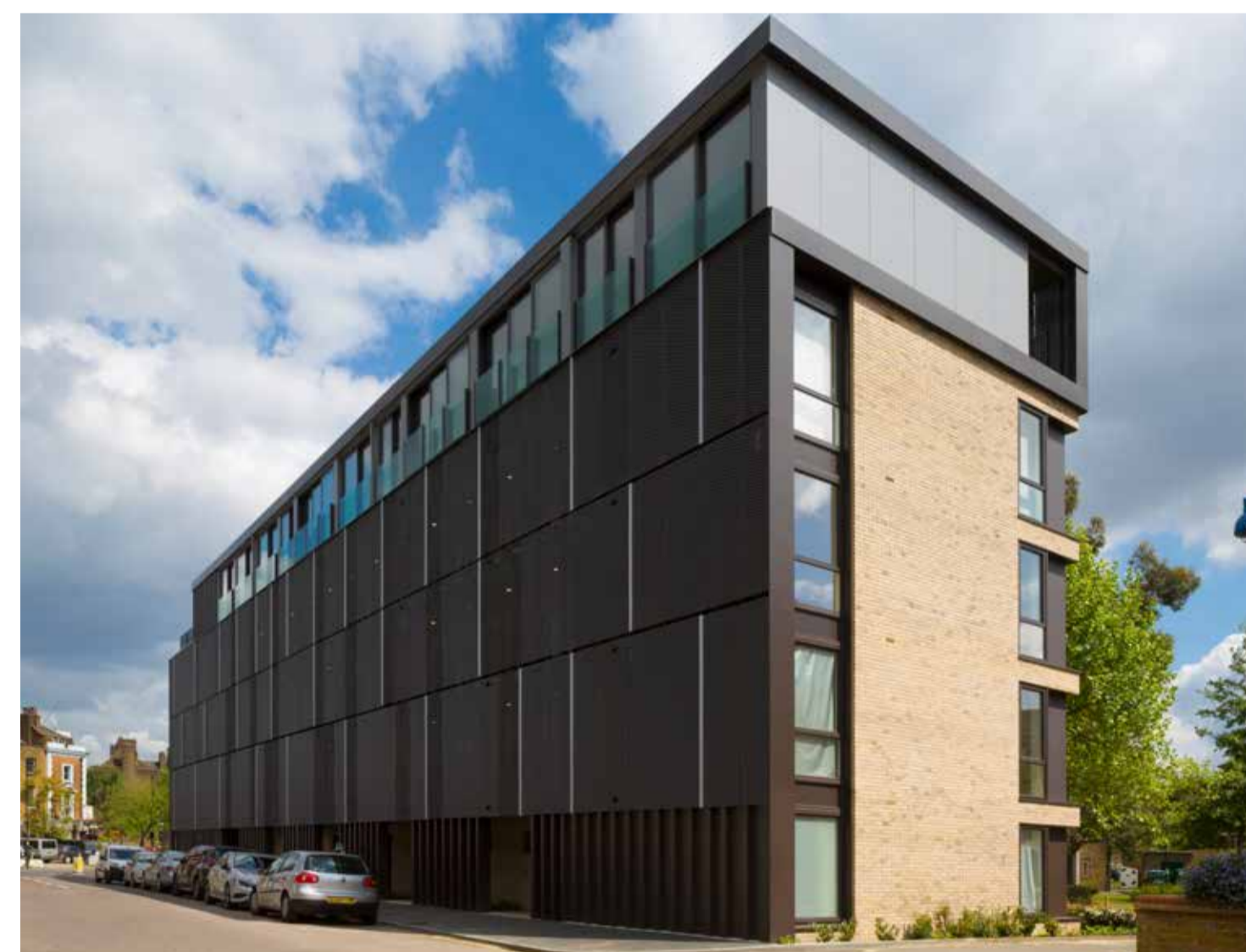
4 - Example of a five-storey residential development with perforated metal panels to fully screen the communal circulation zones
