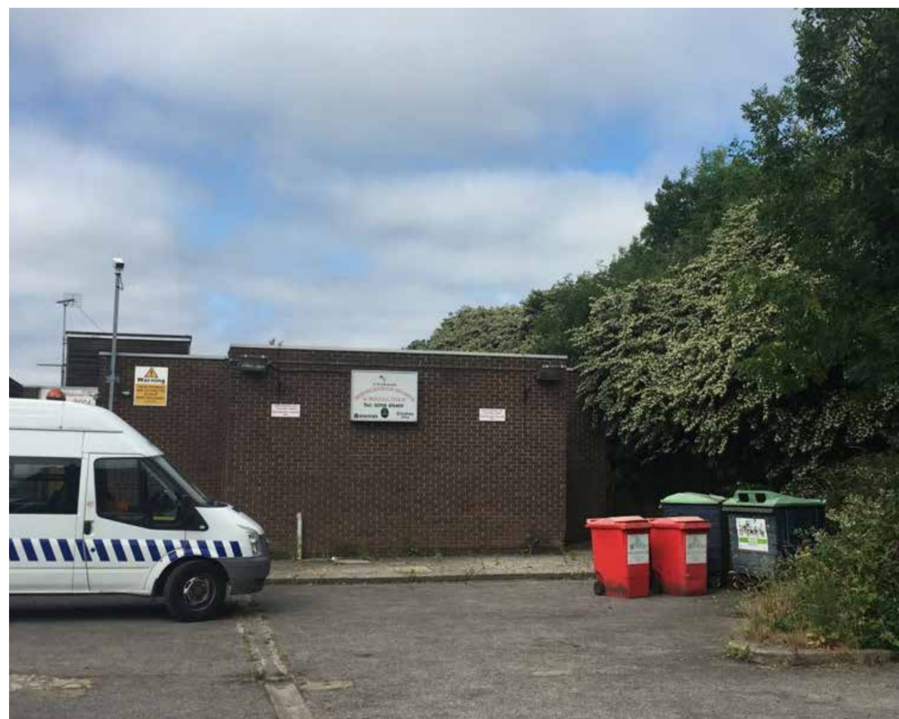
3 - Existing disused members' club on site
