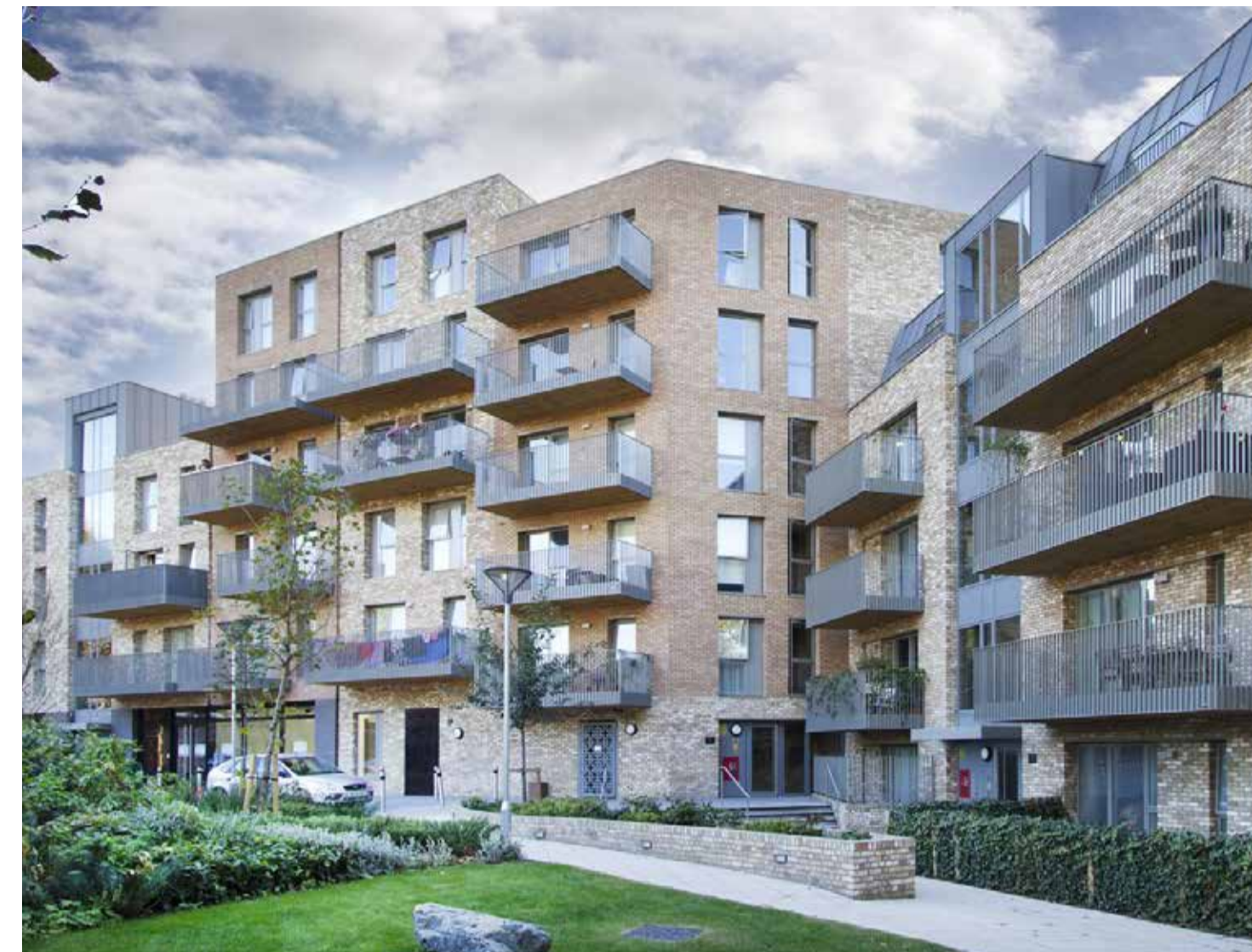
1 - Example of a four/five-storey residential development with complementary tones of brick cladding, projected balconies and generous fenestration
