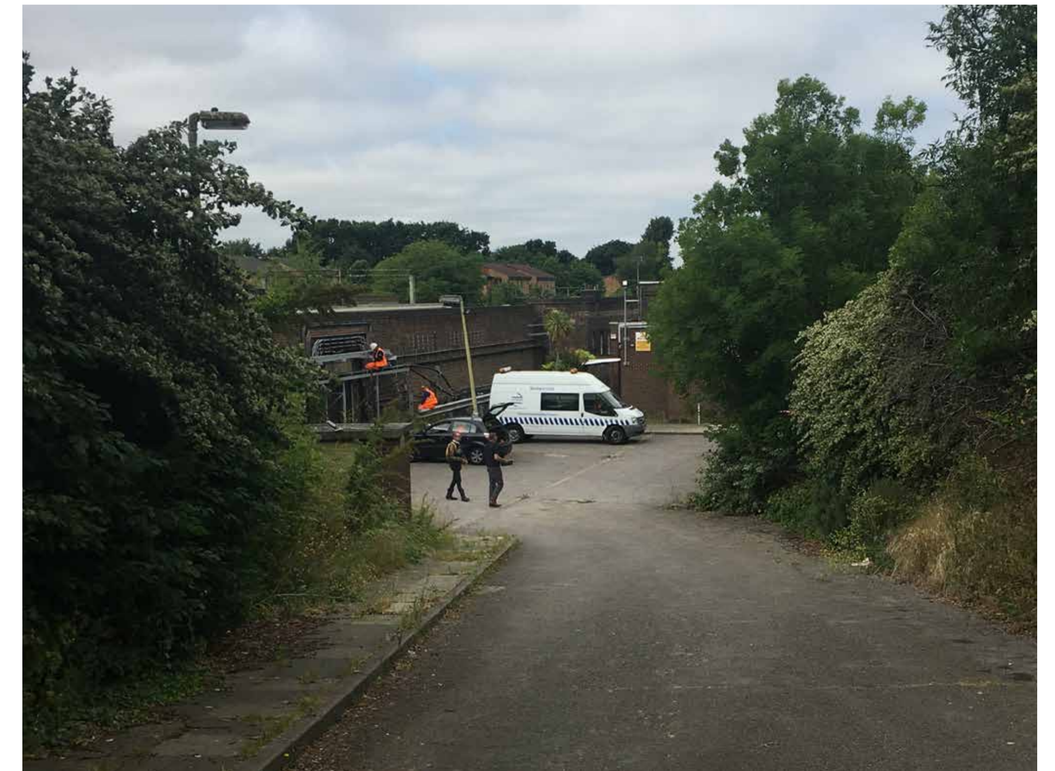
2 - View of the site from the access slope
