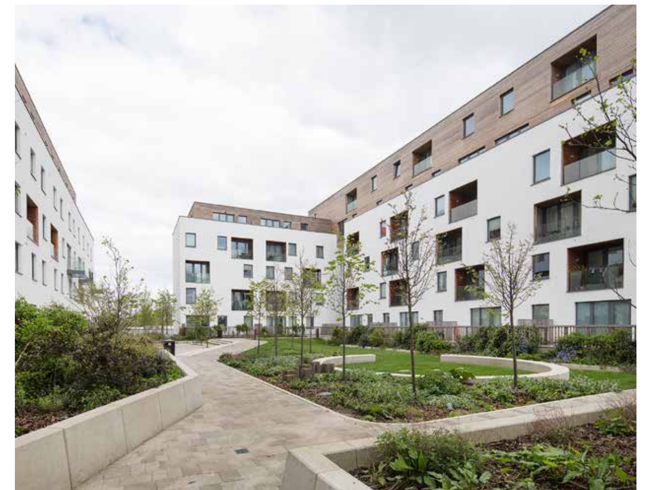
Mixed use development. Apartments, retail, workspace & creche. Colindale, London
