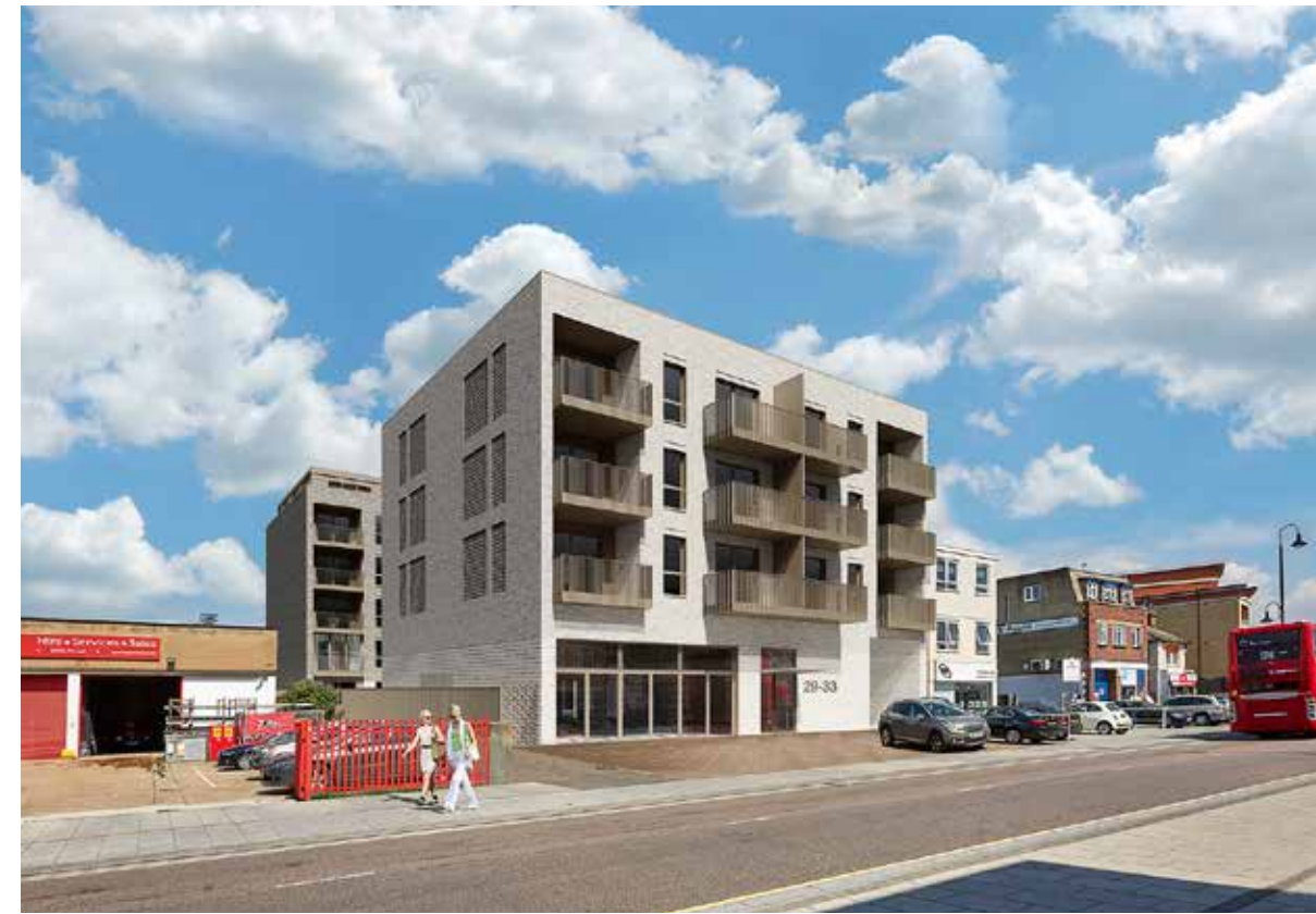
Mixed use development. Victoria Road, Romford. London Borough of Havering
