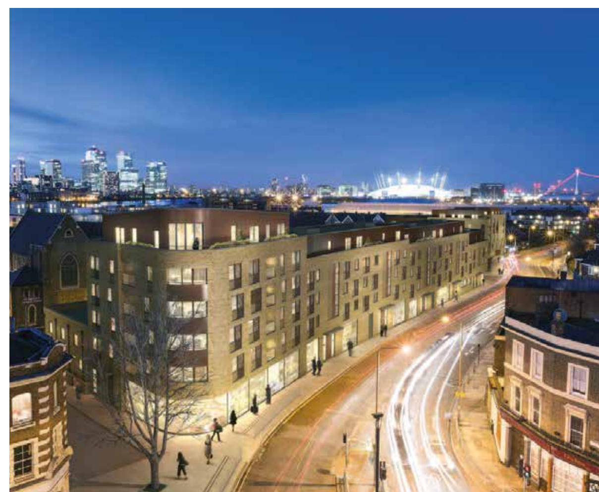
Mixed use development. Residential & retail. Blackwall Lane, Greenwich, London
